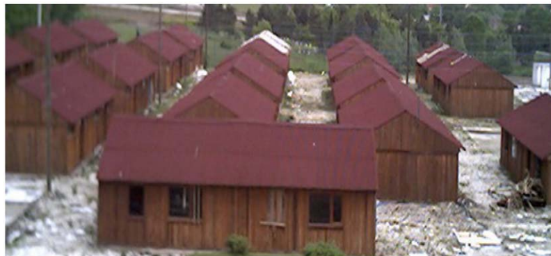
Fig. 1. Beci temporary housing site (general view).
