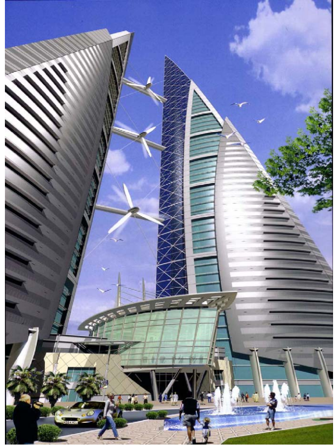
Fig. 1. The Bahrain World Trade Centre. The total built-up area 120,000 m 2 ; Twin Towers-240 m height; 45 useable floors and a shopping mall.
